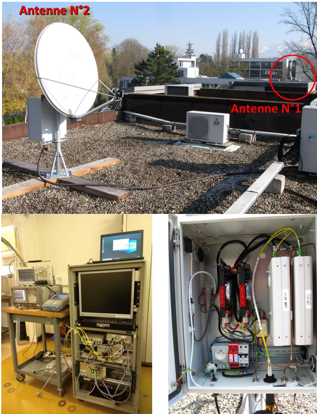
Figure 4: Top: Antennas on the IRAM headquarters roof in Grenoble. Bottom left) Indoor rack of electronics and control pc, Bottom right) Outdoor rack of electronics.
